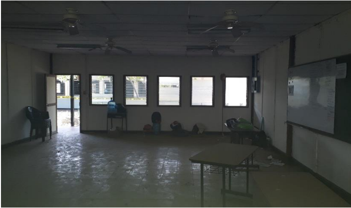
Conditions of the classrooms before remodeling
