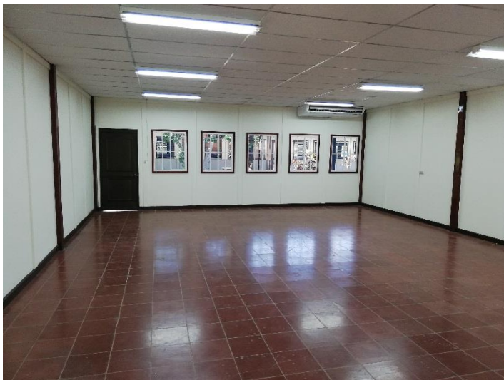
Conditions of the classrooms after the remodeling
